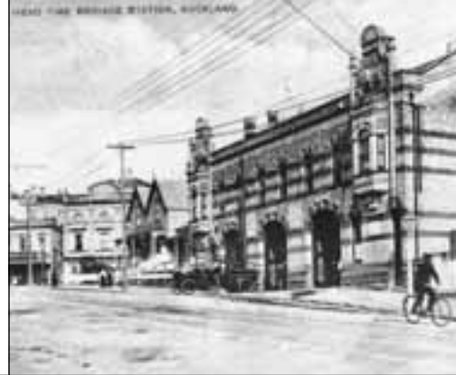
35. Head Fire Brigade Station | 50 Pitt Street
